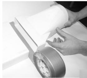
ensuring they are pushed firmly together. Tape the joint ensuring it is central across the tape width.
