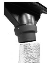
Slide a speed clamp (X332) over the ducting and push-fit the ducting around the 125mm diameter spigot of the terminal pipe adaptor. Tighten the speed clamp to secure.
