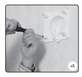
Attach the internal vent housing with 4 screws.
