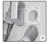
Place the internal butterfly vent arm in the slot.
