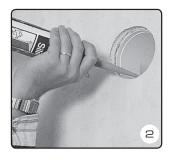
Mount the pipe and seal against the wall, both inside and outside, with for example a sealing agent.
