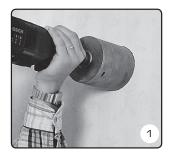
Use a core drill with min. dimension  $\emptyset102mm$  for Fresh 90 and  $\emptyset$  150mm for Fresh 90dB. Drill from inside to outside. Drill the hole so that the pipe slopes slightly downwards.
